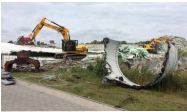
Figure 24 | Oxy-acetylene cutting preparation of tower base
